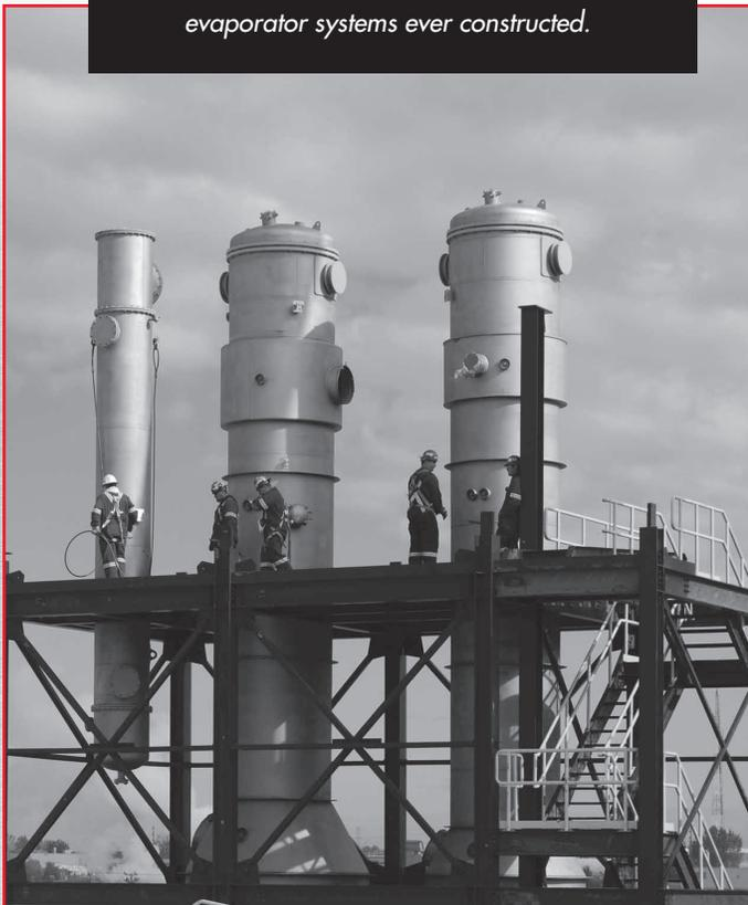
When West Coast Reduction, Ltd made the decision to build a brand new rendering plant for non-SRM beef products at their Alberta Processing Division location in Calgary, one operating criterion took precedence: the new facility had to be energy efficient. The solution: an evaporator system that takes advantage of recycled waste heat from other plant systems to dramatically reduce natural gas consumption.
